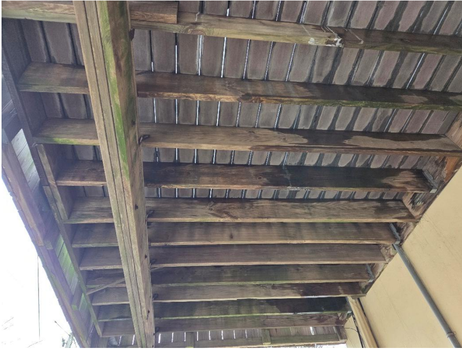
2 nd Floor Deck at 620
