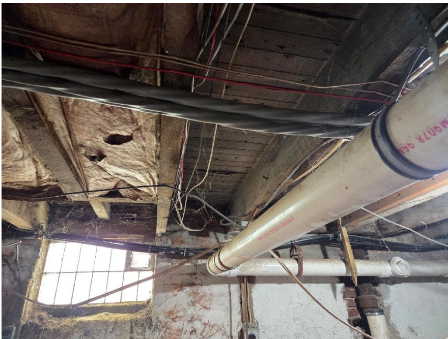
Frist Floor Framing View from basement at 620
