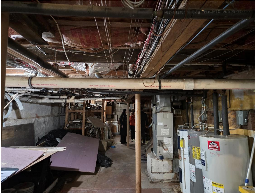
Basement of 620 Looking toward the Front
