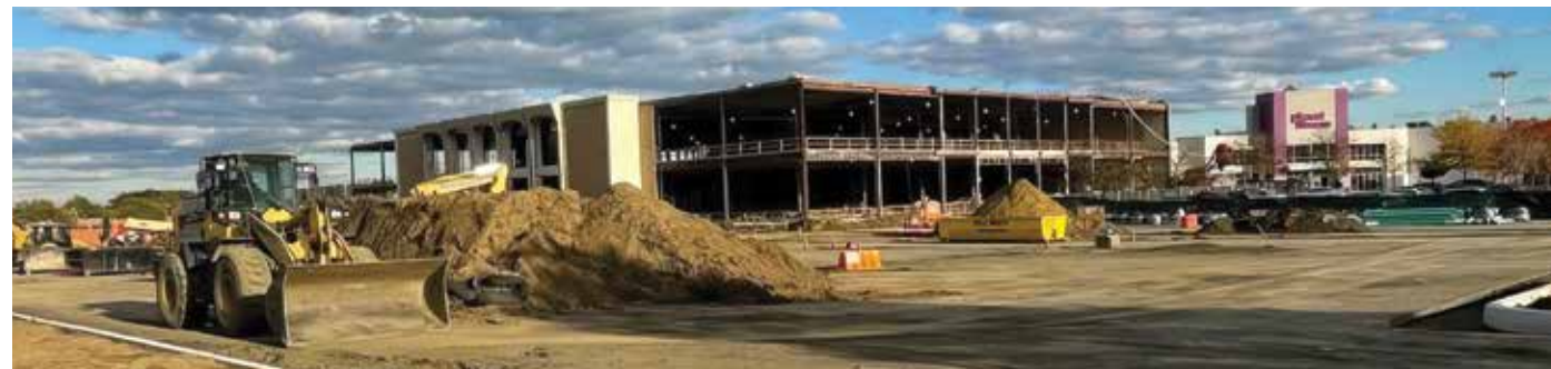
Work progresses at the close of 2022.
