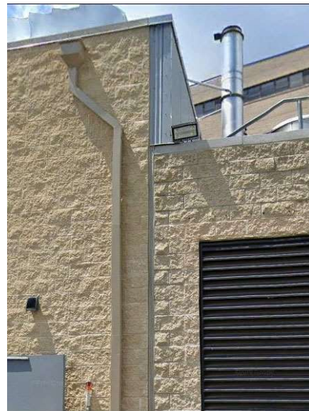
Infill & 1985 Bldg: Split-face Block Masonry Walls
