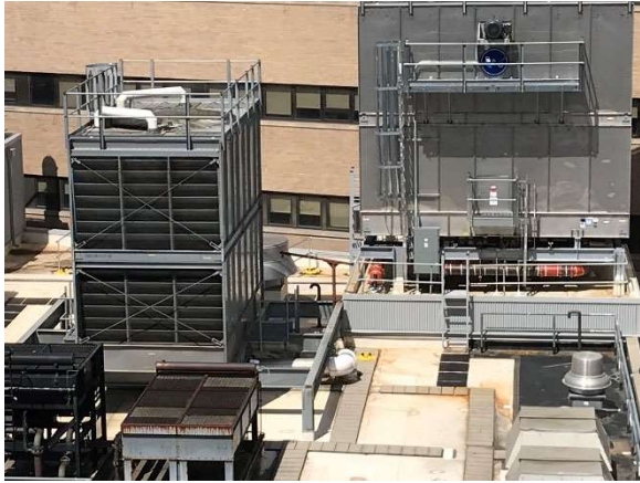
CEP (1985 Bldg) Roof: EVAPCO Cooling Towers
