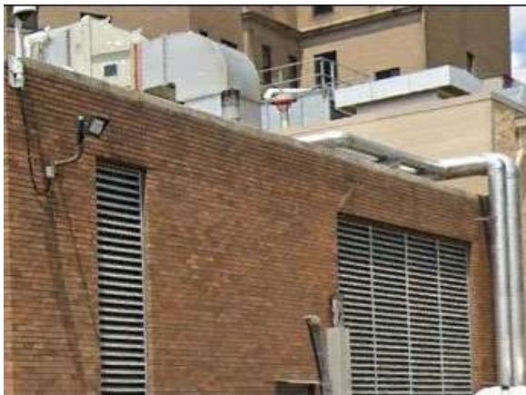
Boiler Plant (East): Older Brick Masonry Walls
