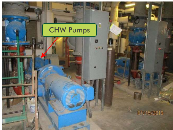
Condenser Water & Primary CHW Pumps
