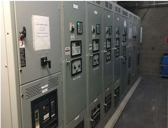
Emergency Paralleling Switchgear
