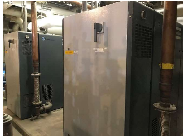
Atlas Copco Medical Air Compressors
