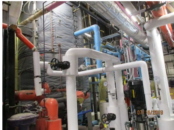
2500-gallon Steam Condensate Surge Tank
