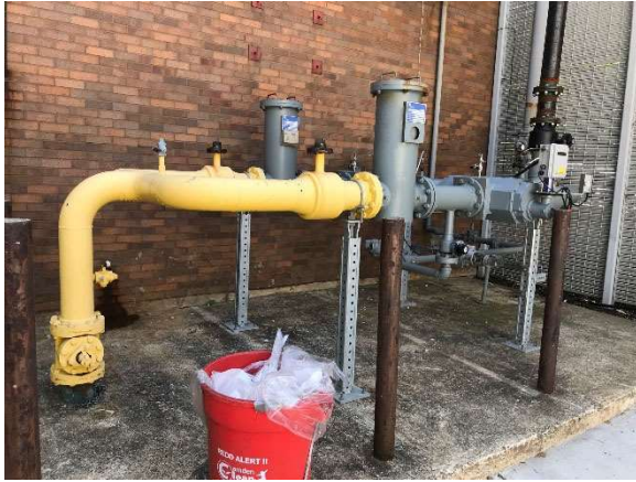
Natural Gas Service for Boilers
