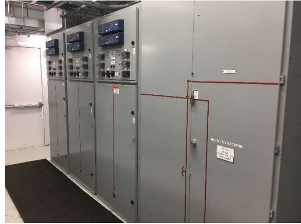
"Service B" Section of 26.4-kV Switchgear
