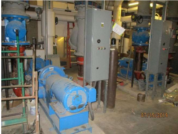
CEP (1985 Bldg): Condenser Water Pumps
