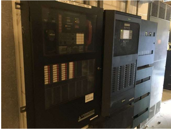
Siemens Fire Alarm Panels
