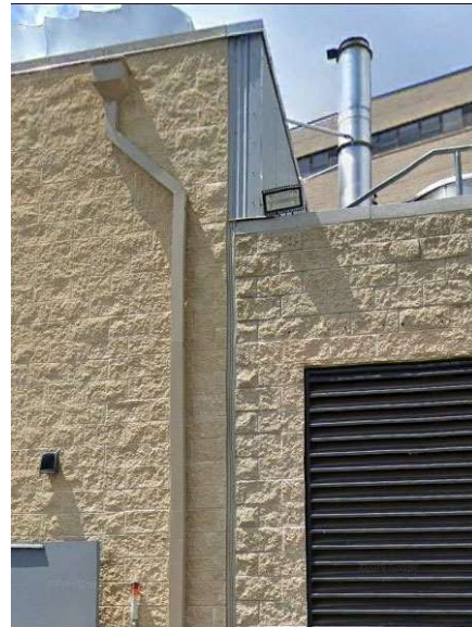
Infill & 1985 Bldg: Split-face Block Masonry Walls
