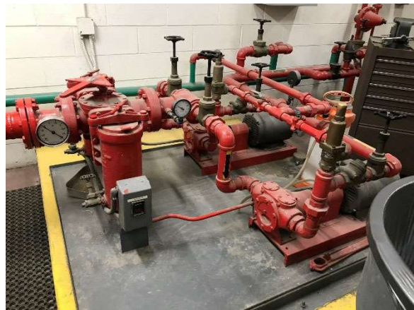
Fuel Oil Pumps Serving the Boilers
