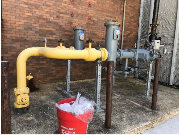
Natural Gas Service for Boilers
