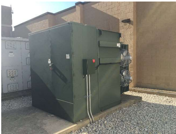
26.4-kV to 13.2-kV Transformer
