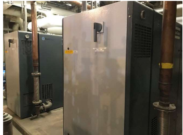
Atlas Copco Medical Air Compressors
