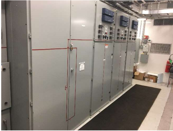
"Service A" Section of 26.4-kV Switchgear
