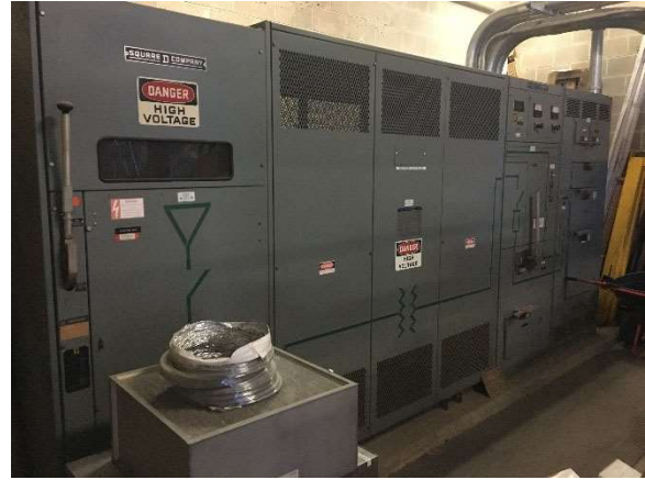
1985 Bldg: Unit Substation
